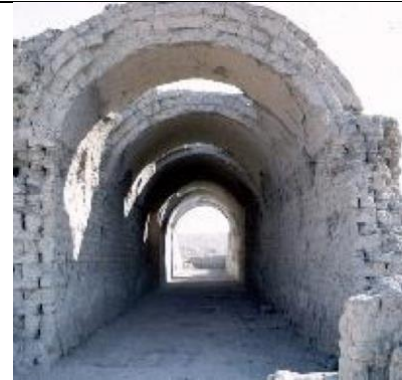
Mud brick vaults that form the Ramesseum.
