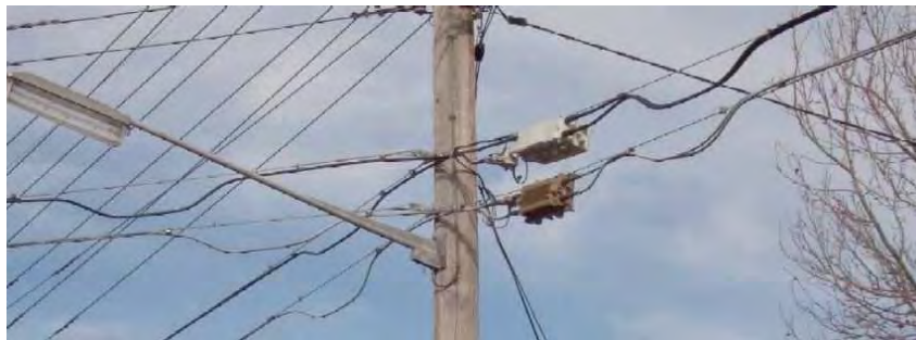
HFC cable on power poles in a suburban street
